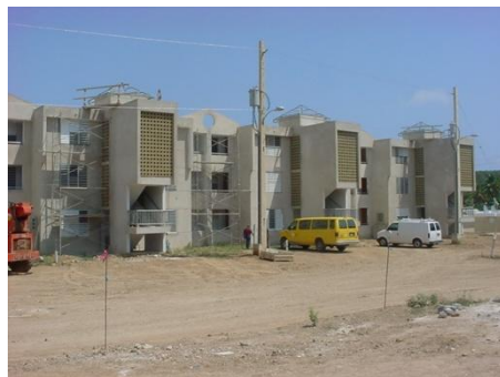
Partial view of 30 houses under construction
