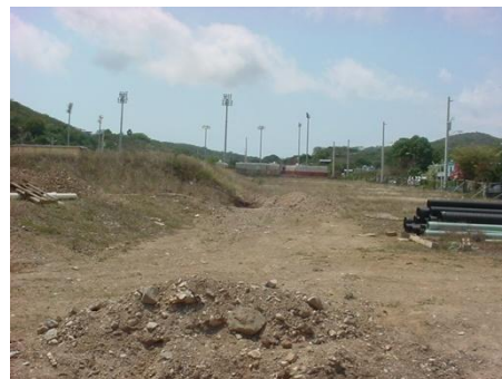
Partial view of site for construction of 102 housing units
