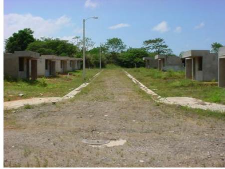
Partial view of 16 houses under construction
