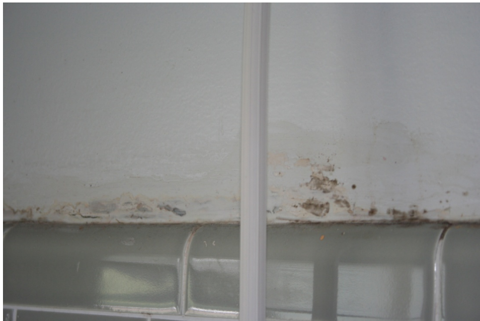
Unit 11: Mold protruding from wall through paint and peeling in bathroom.
