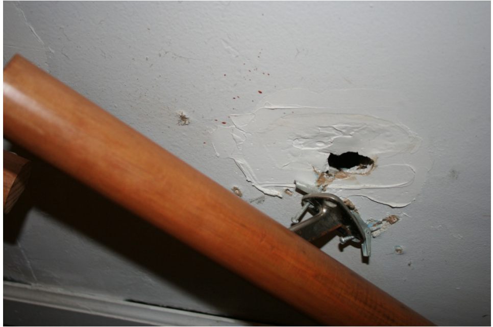
Unit 22: Damaged wall due to insecure handrail at second floor stairs.
