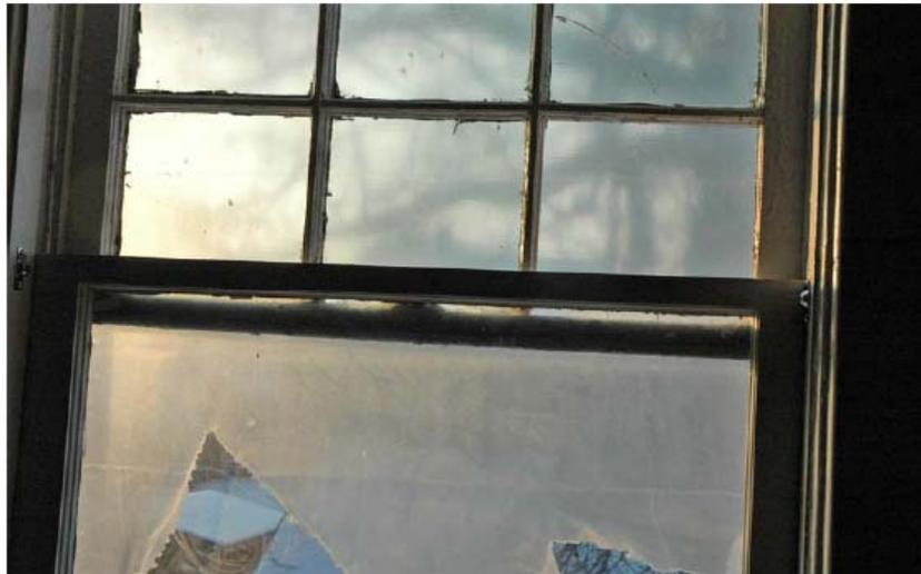
Household 7614: A large gap between the top of the window and the window frame was filled with fibrous material and allowed air filtration. A window pane in a young (5 years old) child's room was broken.
