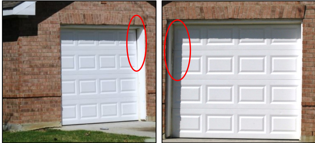
Figure 1: The garage door had a gap between the door and the right side trim. Minor damage was noted on the top right side of the bottom panel. The trim on the left side appears to be rotted.
