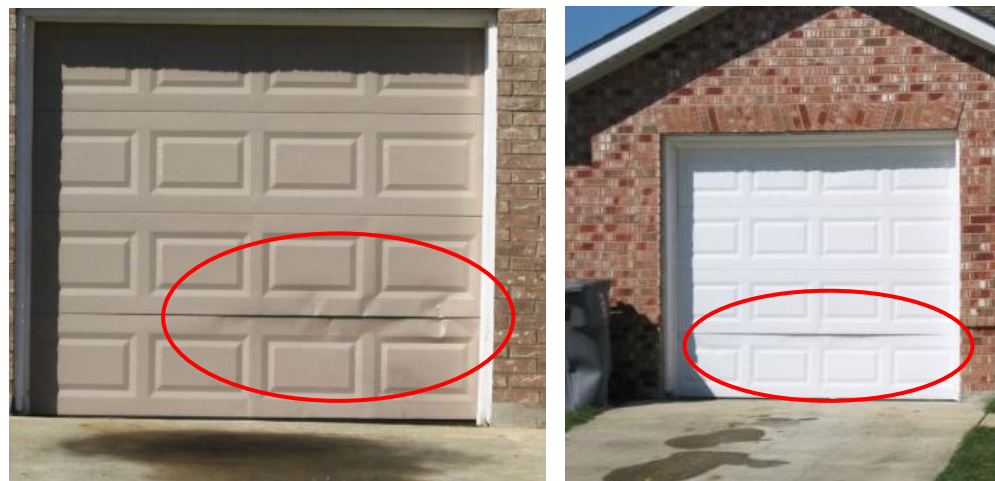
Figure 2: These garage doors appear to have been properly installed; however, they have been damaged.
