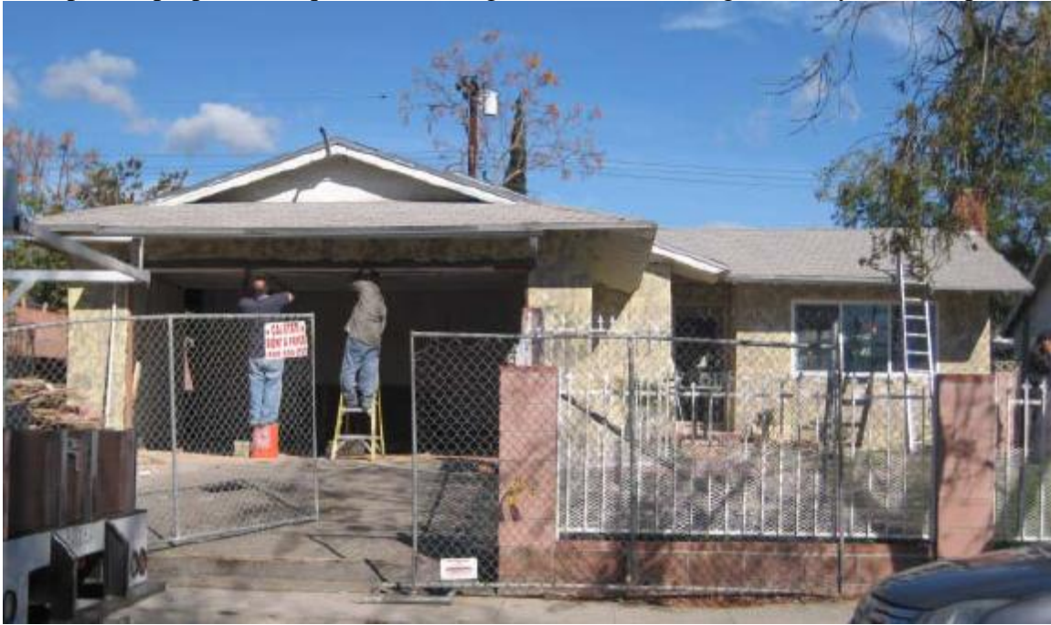
Examples of properties acquired and being rehabilitated through the City's subrecipient.
