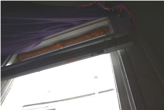
Exposed insulation at top of window.
