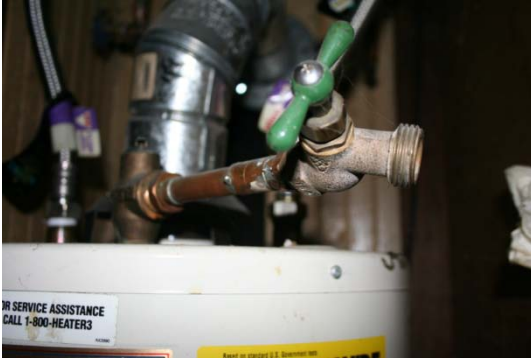
Water heater with improperly blocked pressure relief valve.
