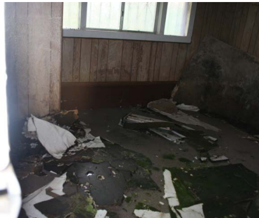
Missing door to abandoned room located adjacent to occupied housing unit resulting in potential fire and safety hazard.
