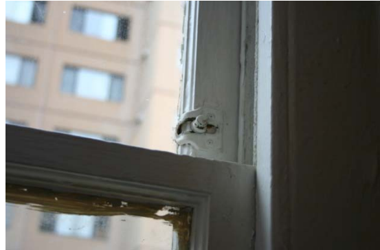
Affixed window side safety lock not removable hindering tenant's ability to access the adjacent fire escape in the event of an emergency.
