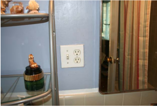
Missing GFCI outlet in updated bathroom of housing unit.
