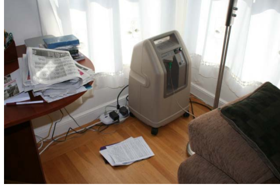
Reversed electrical polarity throughout housing unit posing potential safety hazards for occupant using electrical items such as oxygen machine.
