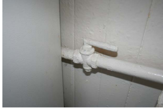
Gas valve painted shut hampering the ability to open/close in the event of emergencies.
