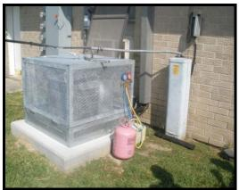
Picture 2 – Kelly Terrace, Unit 82: Outdoor condenser unit installed as well as concrete slab with steel cage and line runs. Testing of some of the HVAC installations was visibly in progress.
