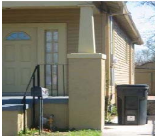
Right side view of property’s exterior.
