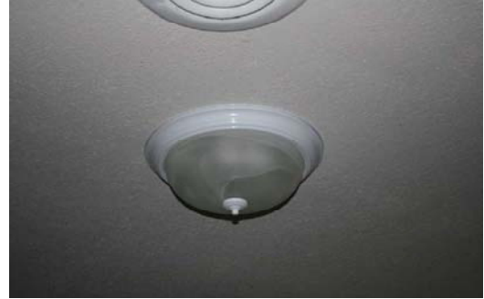
Picture 2: New Energy Star light fixture installed at Ridgeland Terrence in Blue Mountain, MS
