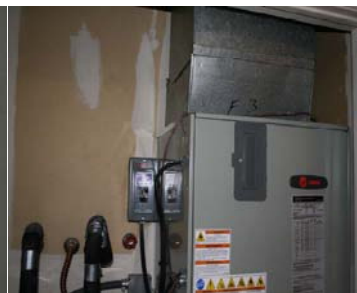
Picture 4: Air handler and condensing coils
