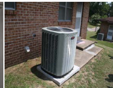
Picture 5: Trane heat pump compressor
