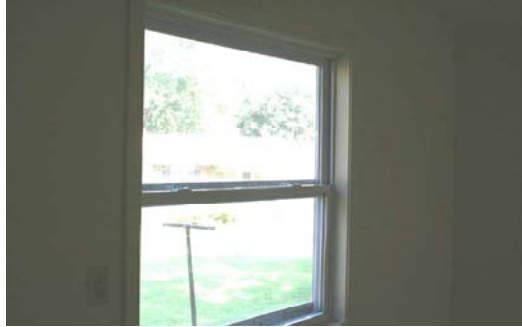
Picture 1: New window installed at Willow Terrence in Corinth, MS
