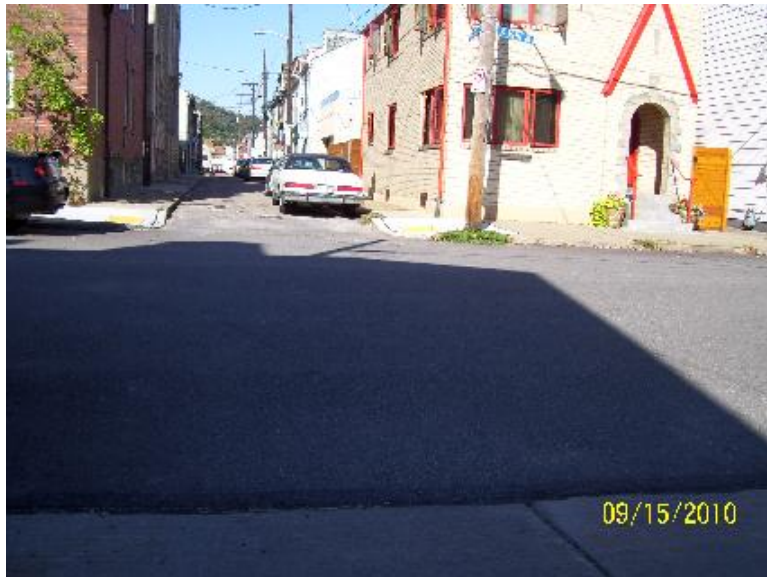
Resurfacing of South 19th Street (completed)
