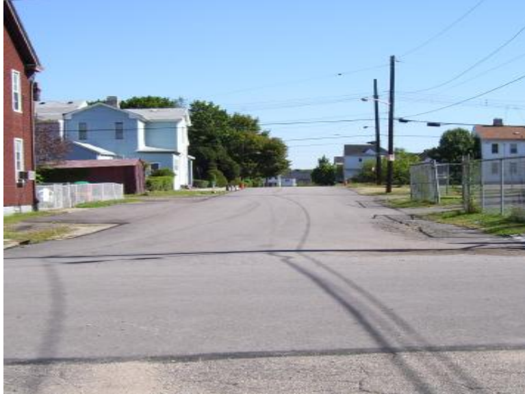
Resurfacing of Ashley Street (completed)
