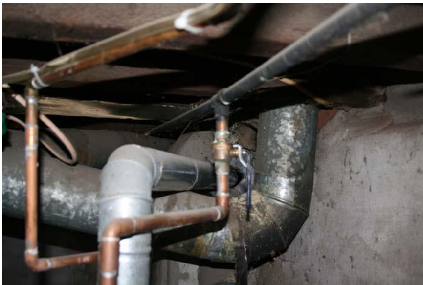
The water heater flue pipe level needs to have a positive slope for fumes to escape.
