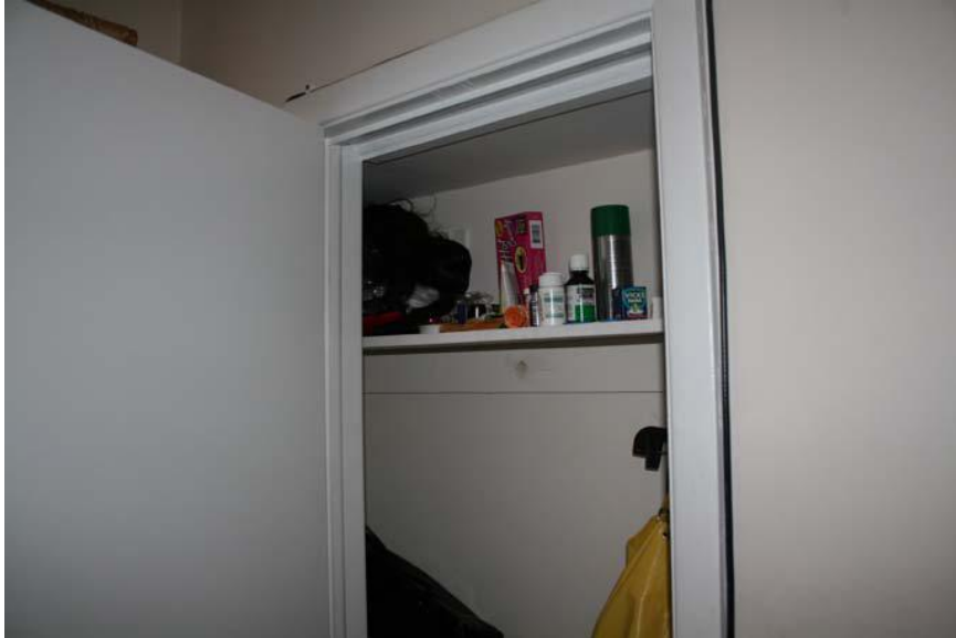
The closets in bedrooms 2 and 3 are only 14.5 inches deep.
