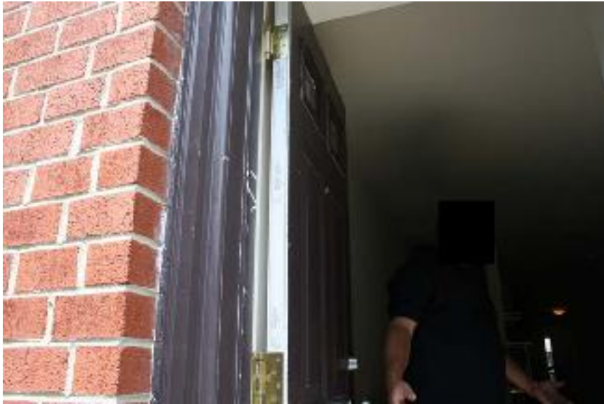
The contract required 90-minute fire rated doors. Doors in 5 of 10 units inspected were only fire rated for 20 minutes. Note: We shielded the identity of the inspector.
