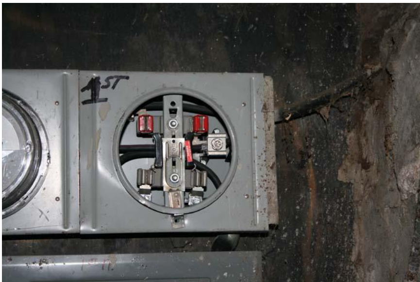
The meter base is not secured for the first floor. The tenant has access to the basement. Exposed terminals are a 24-hour exigent health and safety violation. HUD informed us that the Authority corrected the issue after the inspection.
