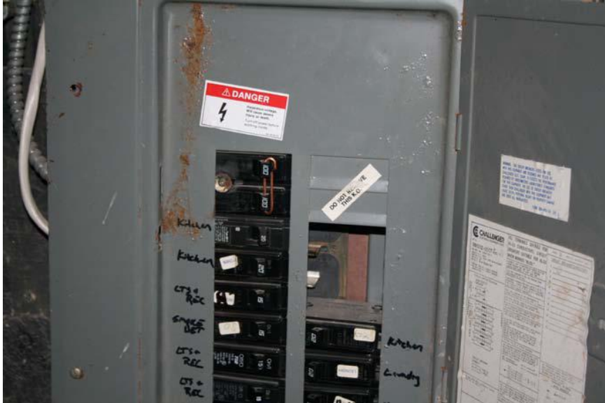
There are open slots in the breaker panel in the basement. This hazard is a 24-hour exigent health and safety violation. HUD informed us that the Authority corrected the violation after the inspection.
