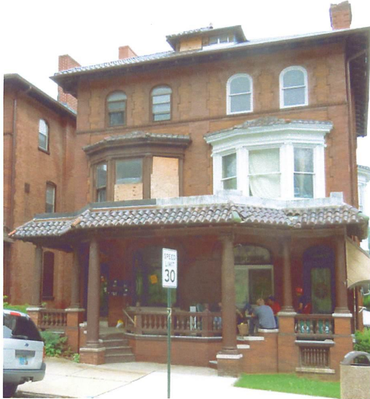
1602 Mineral Springs Road, Reading PA, (on the left) for which rehabilitation specifications are being developed prior to obtaining bids and starting renovation work.
