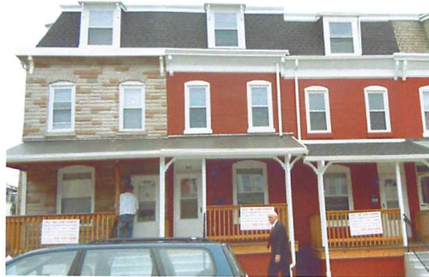
661, 663, and 665 Tulpehocken, Reading PA; two of these fully rehabilitated houses now ready for sale were used to compare construction costs
