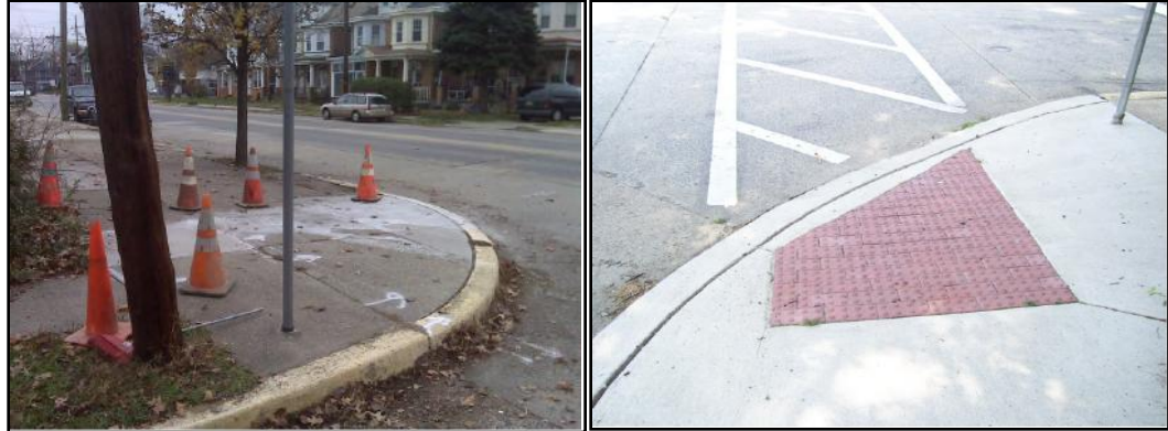
Before (left) and after (right) pictures illustrate the installation of curb cuts along Haddon Avenue in Collingswood (completed).
