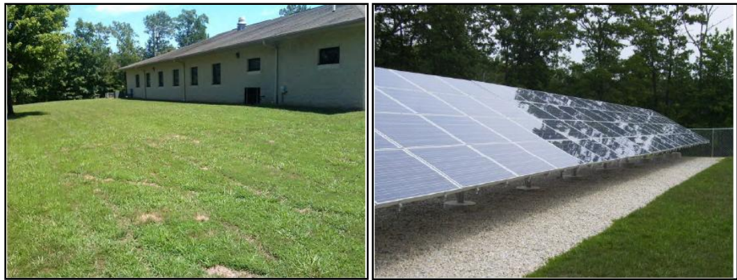
Before (left) and after (right) pictures illustrate the installation of a solar panel system at the Winslow Township senior center (completed).
