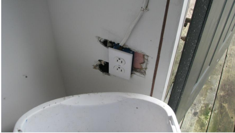
Hole in wall at electrical outlet and exposed wiring not in conduit that the Authority failed to report on its previous inspection.
