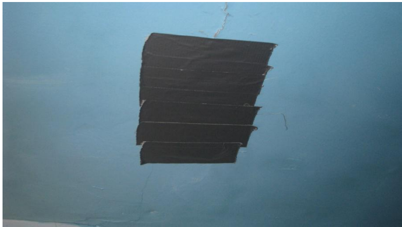
Leaking bathroom ceiling patched with tape by tenant.
