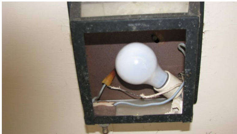
Exposed wiring on an exterior light fixture that the Authority failed to report during its previous inspection.
