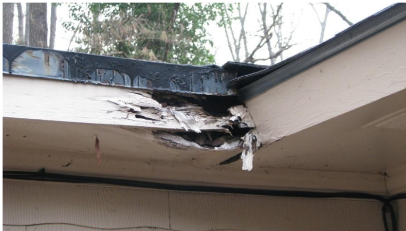
Rotting soffit that the Authority failed to report on its previous inspection.
