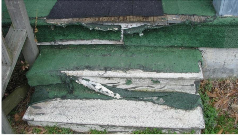
Tripping hazard caused by unsecured carpet on front porch/steps.
