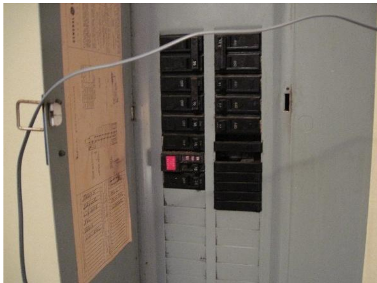
Two Missing breakers on right side of panel leaves high voltage wiring exposed
