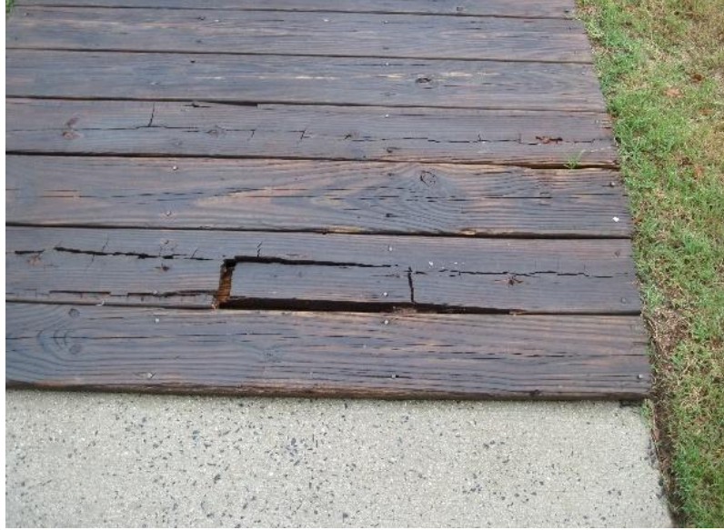
Badly deteriorated ramp creates tripping/falling hazard
