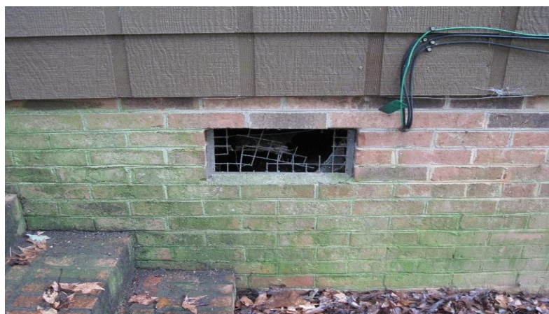
Badly damaged foundation vent allows easy entry of vermin
