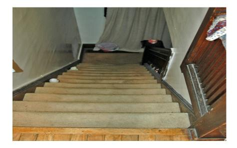
Household 1014364: The stairway to the basement needs to have a handrail that extends the entire length of the stairway.
