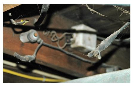
Household S064675: A live abandoned wire on the basement ceiling has exposed contacts at the ends.
