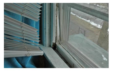
Household 1021560: The window doesn't lock because the sash is too large for the window frame and doesn't line-up for the locks.
