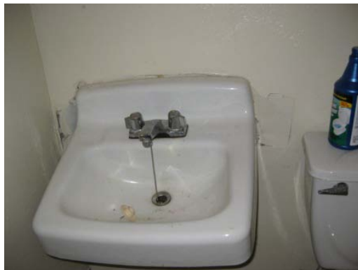
Picture 7: Unit 107. The wall behind this sink was severely damaged. It was unclear who was responsible for the damage.
