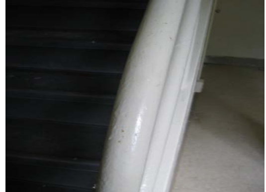
Picture 8: Unit 48. This handrail had paint drippings and rust appeared to have bled through the paint.
