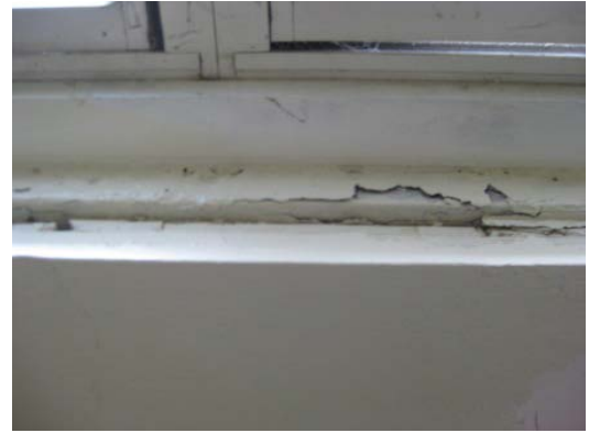
Picture 6: Unit 48. The chipped paint indicated that the contractor had not cleaned or encapsulated the window frame as required.
