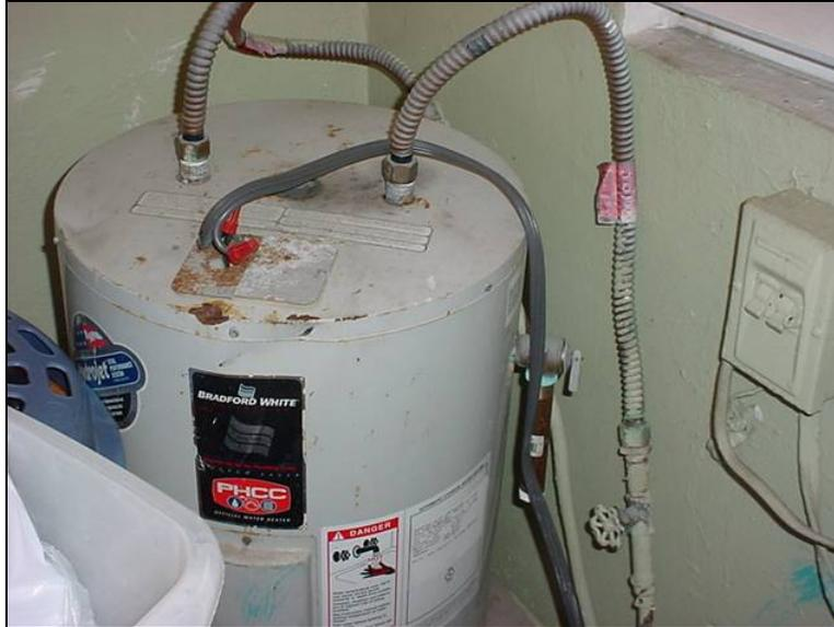
Improper wiring of water heater with exposed wire connections, creating an electrical shock hazard. In addition, the pressure relief valve discharge pipe was too short. This deficiency was not reported by the authority during its August 23, 2007, inspection.
