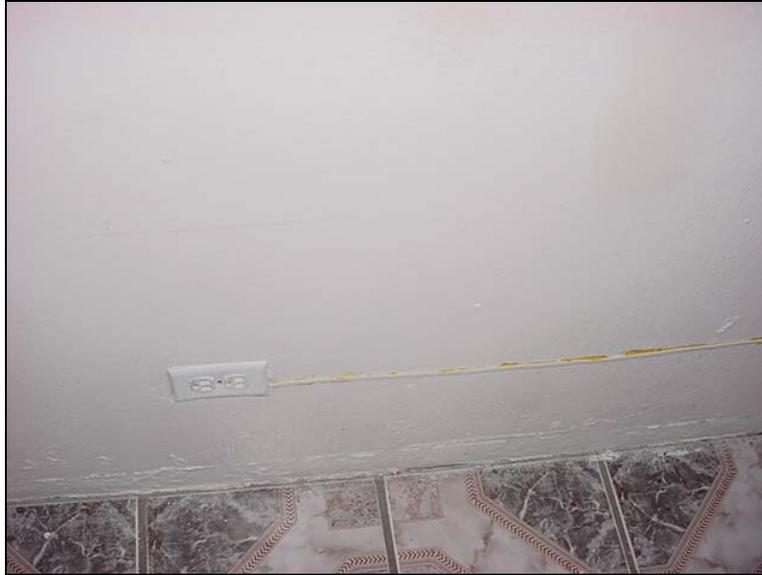
Electrical outlet improperly wired and unshielded electrical wires. This deficiency was not reported by the authority during its September 7, 2007, inspection.
