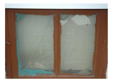
Project #8114: Newly installed window not appropriately sealed and not preventing moisture from entering window perimeter.
