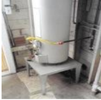
Water heater may not meet code requirements 10
