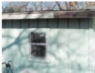
Unpainted roof repair
