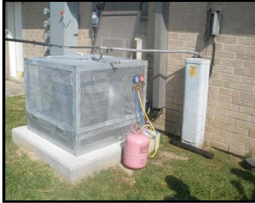
Picture 2 – Kelly Terrace, Unit 82: Outdoor condenser unit installed as well as concrete slab with steel cage and line runs. Testing of some of the HVAC installations was visibly in progress.
